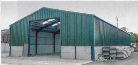
Expansion at Graham Heath Construction means the company can deliver steel-framed buildings to customers in just eight weeks.
